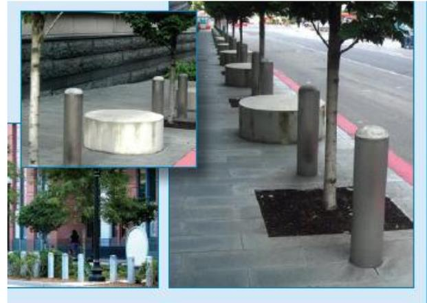
Figure 10.14 – Bollard and Tree Site Barrier.
